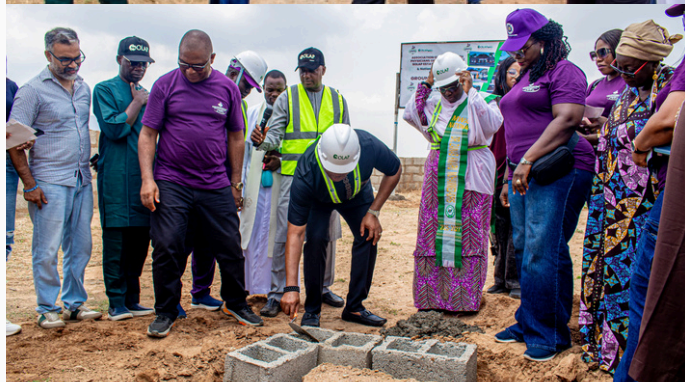
Ground breaking Ceremony/ Foundation laying of the National Secretary by High Chief Mike Duru Ejiogu FCICN, Onowu Igbo Land, CEO, CITYGATE GROUP
